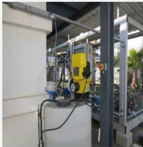
Figure 7. Pump for flux enhancer addition.
